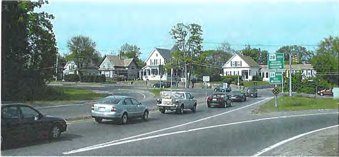
Well-Maintained Houses on Rte. 28 in Path of Any Prospective Alignment, Limiting Opportunities to Extend Harrison Blvd. to the East.
