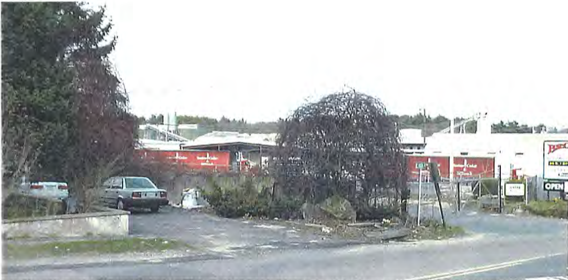
Minimal Greenbelt between Residential and Industrial Districts along East High Street; Roughly 30’ Wide, but Not 7-foot High and “Sight Impervious.”
