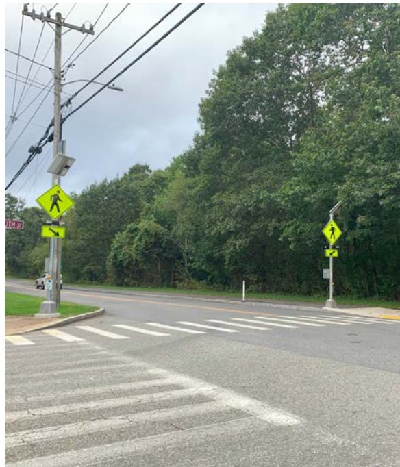
Figure 10-6. Some crosswalks, particularly near schools and along Central Street, have been improved in Avon to include flashing safety beacons and other countermeasures to make crossing the street safer.
