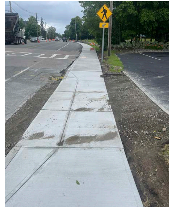
Figure 2.12. Sidewalk improvements underway
