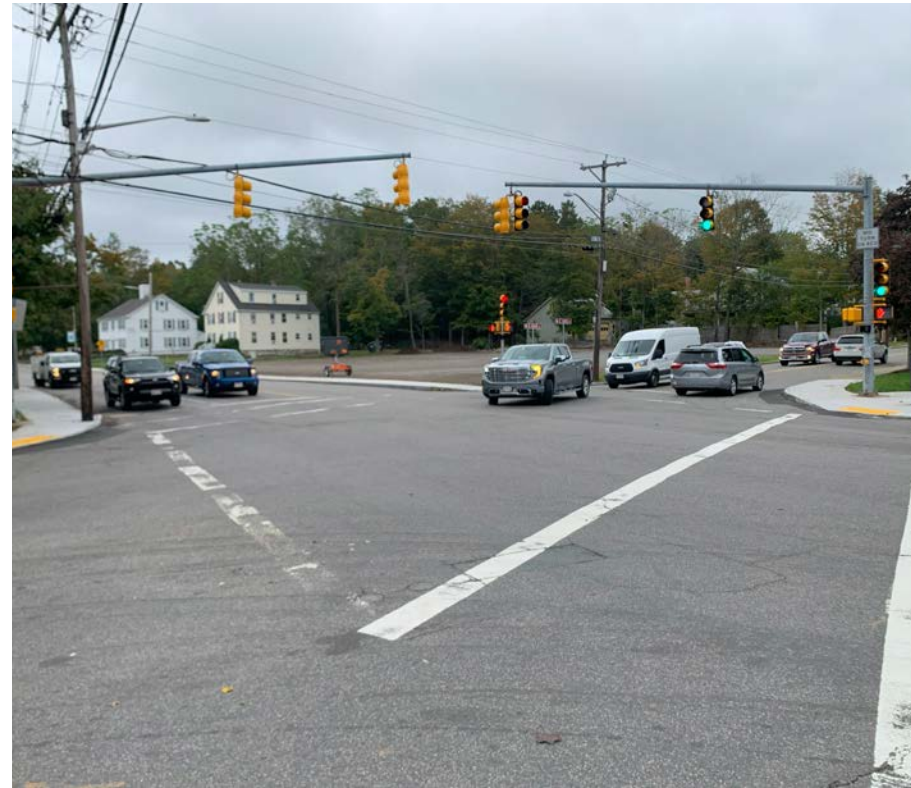
Figure 10-1. The downtown intersection of Main Street (Rt. 28) and High Street is characterized by ample vehicle capacity and traffic, with minimal accommodation for people walking.
