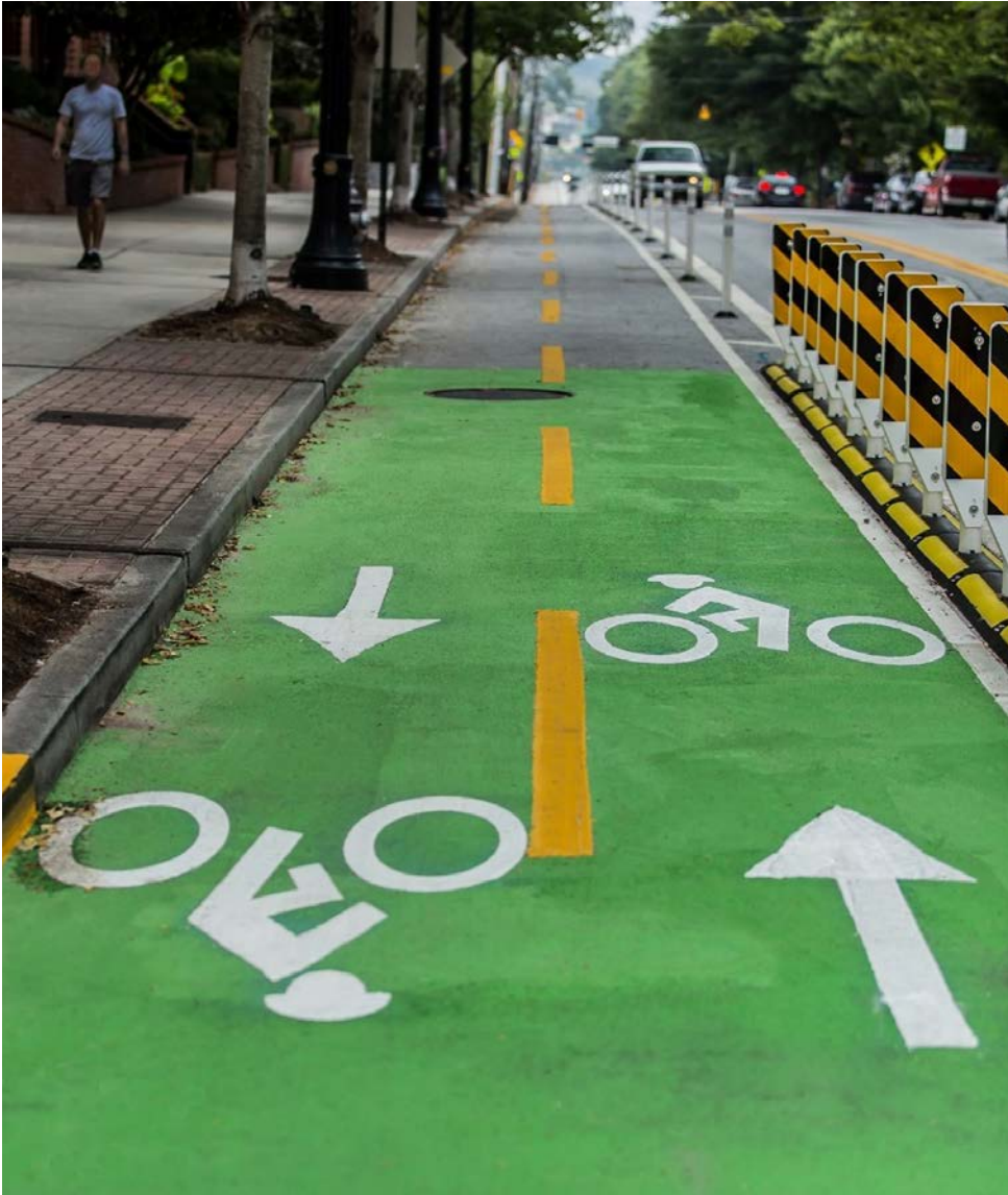
Figure 10-11. A two-way on-street cycle track installed in Jersey City NJ has not only provided space for micro-mobility device users, it has also helped diet a busy arterial to reduce speeds and improve walk safety.
