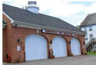
The existing fire department building
